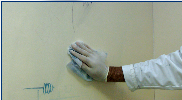
Graffiti removal in progress
